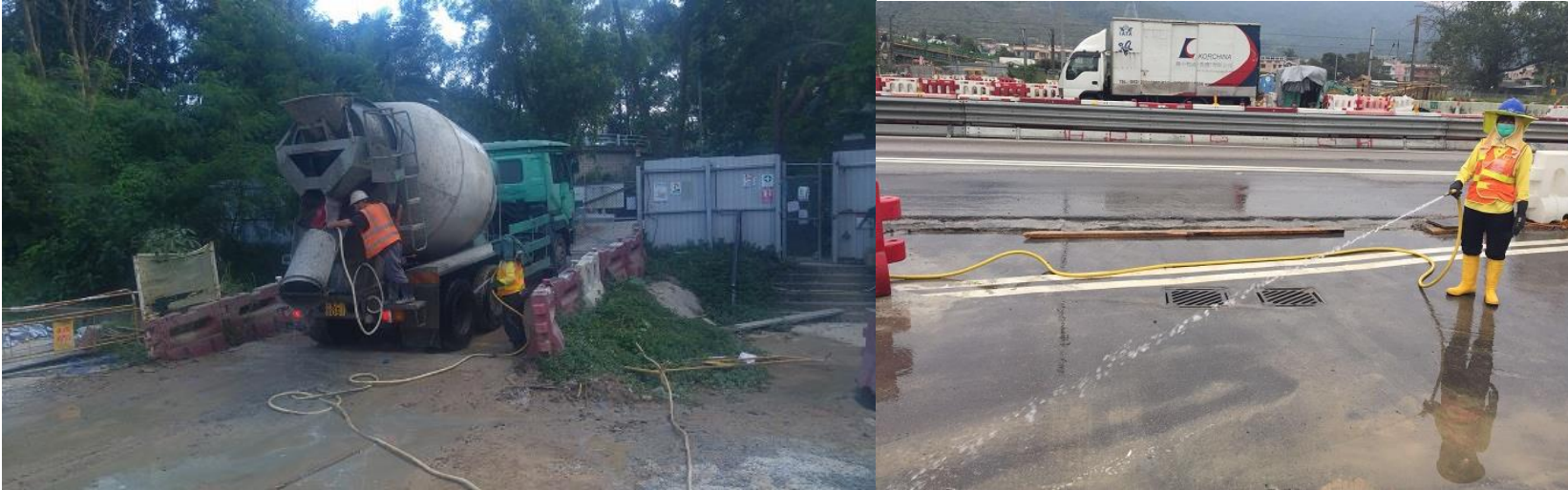
Figure 4 – Wheel Washing Facility at Exit Point
