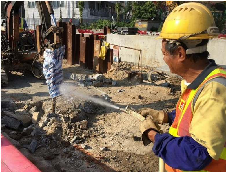
Figure 5 – Water Spray for Dust Emission Construction Activity
