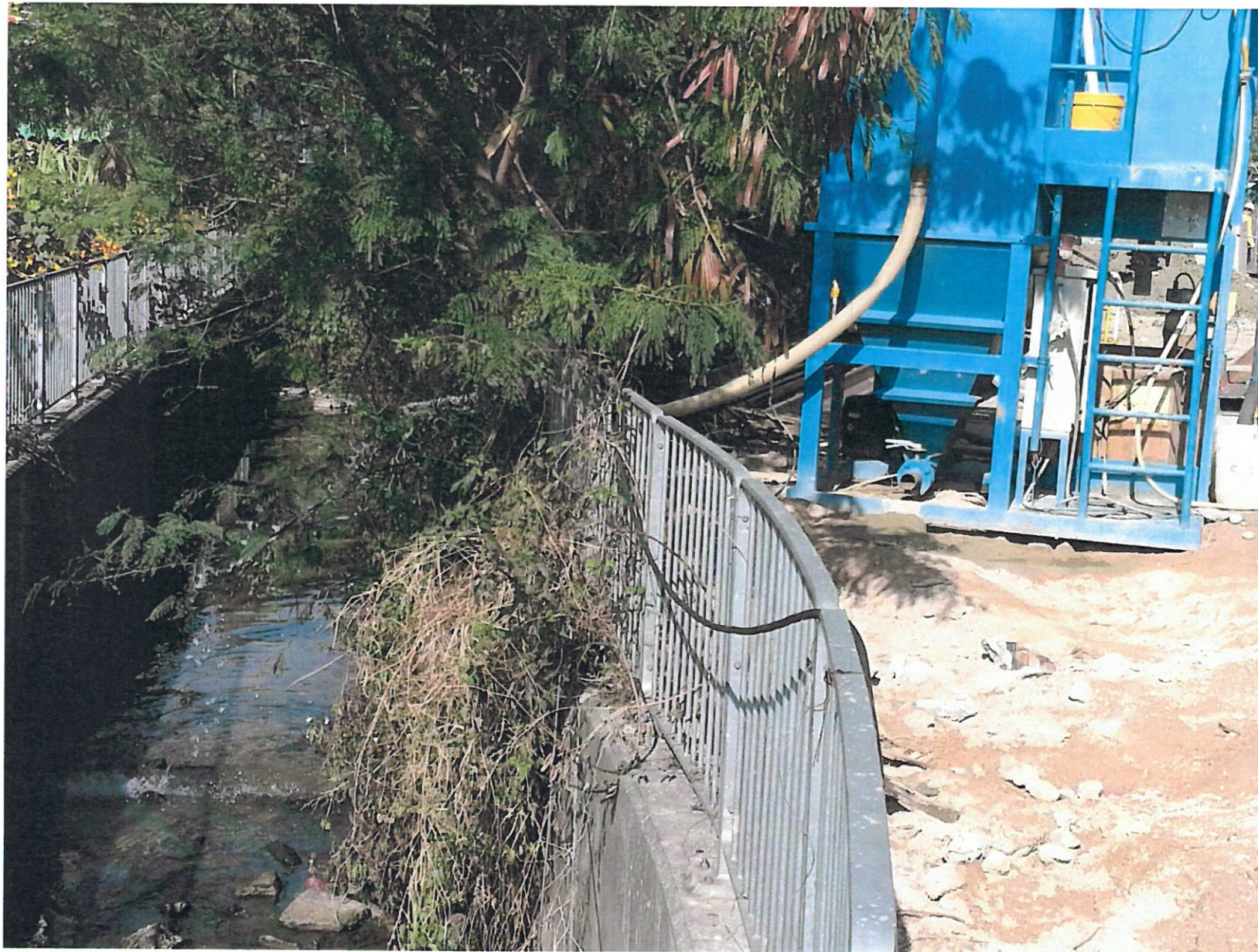
Figure 3 – Photo showing the effluent discharged from the wastewater treatment unit (3 January 2015)
