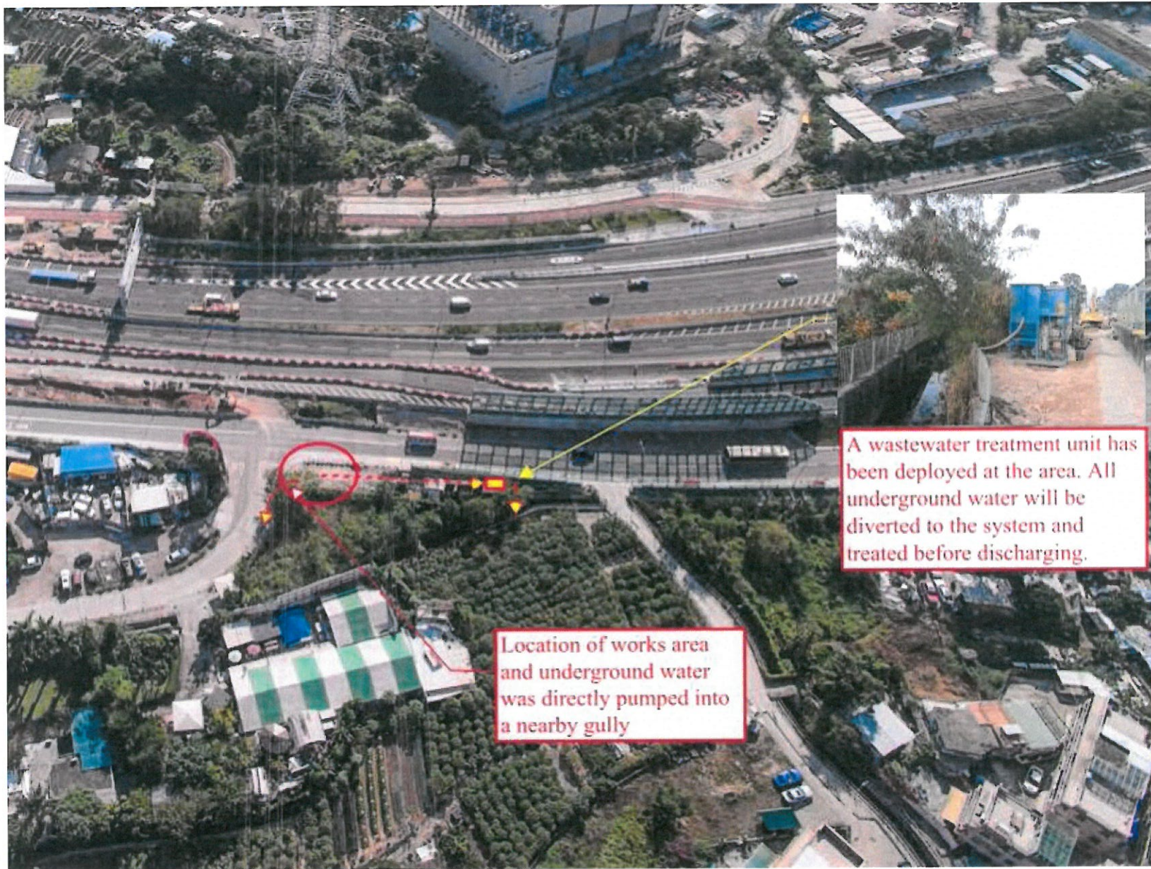
Figure 2 - Installation of the wastewater treatment unit for the complained area
