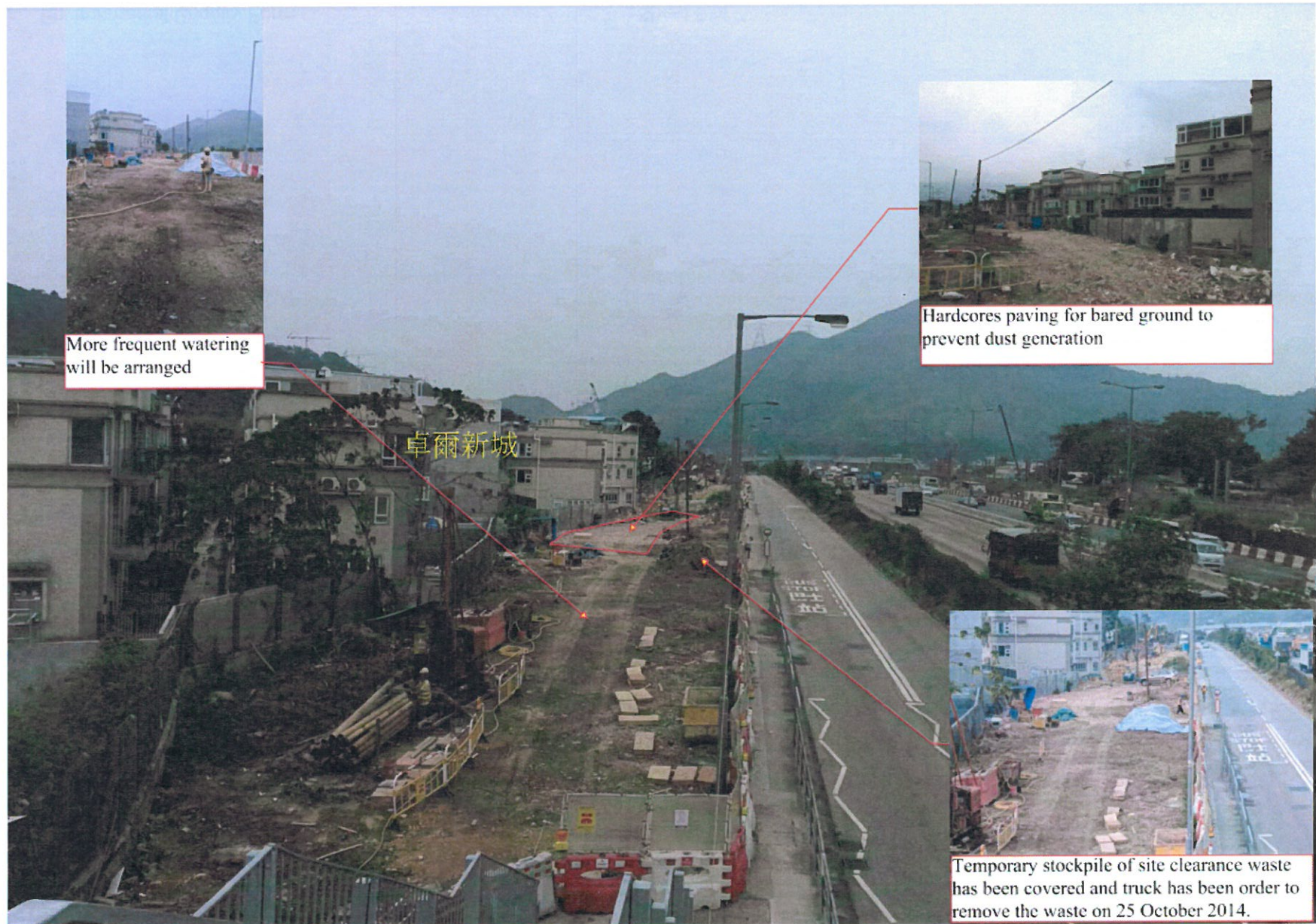
Figure 3 – Dust Suppression Measures
