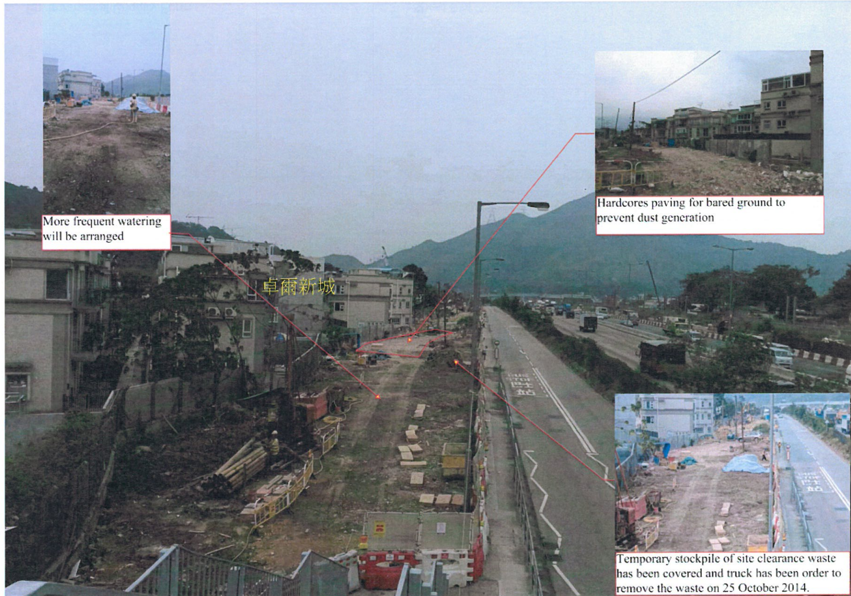
Figure 3 – Dust Suppression Measures
