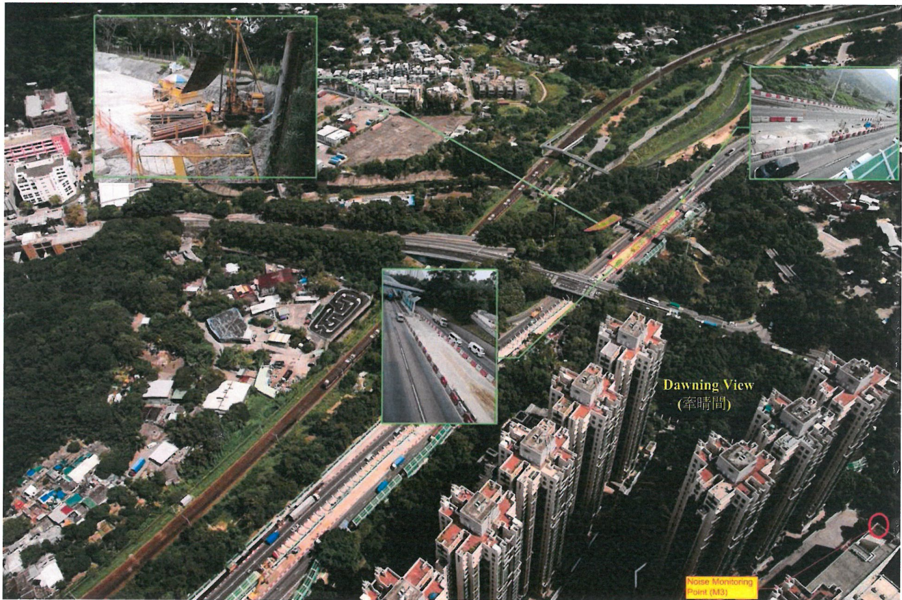
Figure 1 - The location of construction works on 18 June 2014 near the noise monitoring location M3: Wo Hop Shek Pedestrian and Cyclist Bridge
