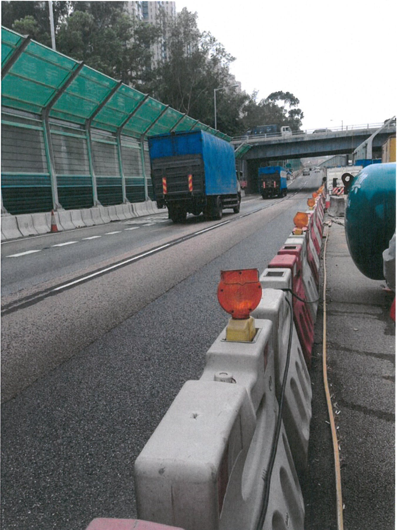
Figure 3 – The works area screened by existing noise barriers
