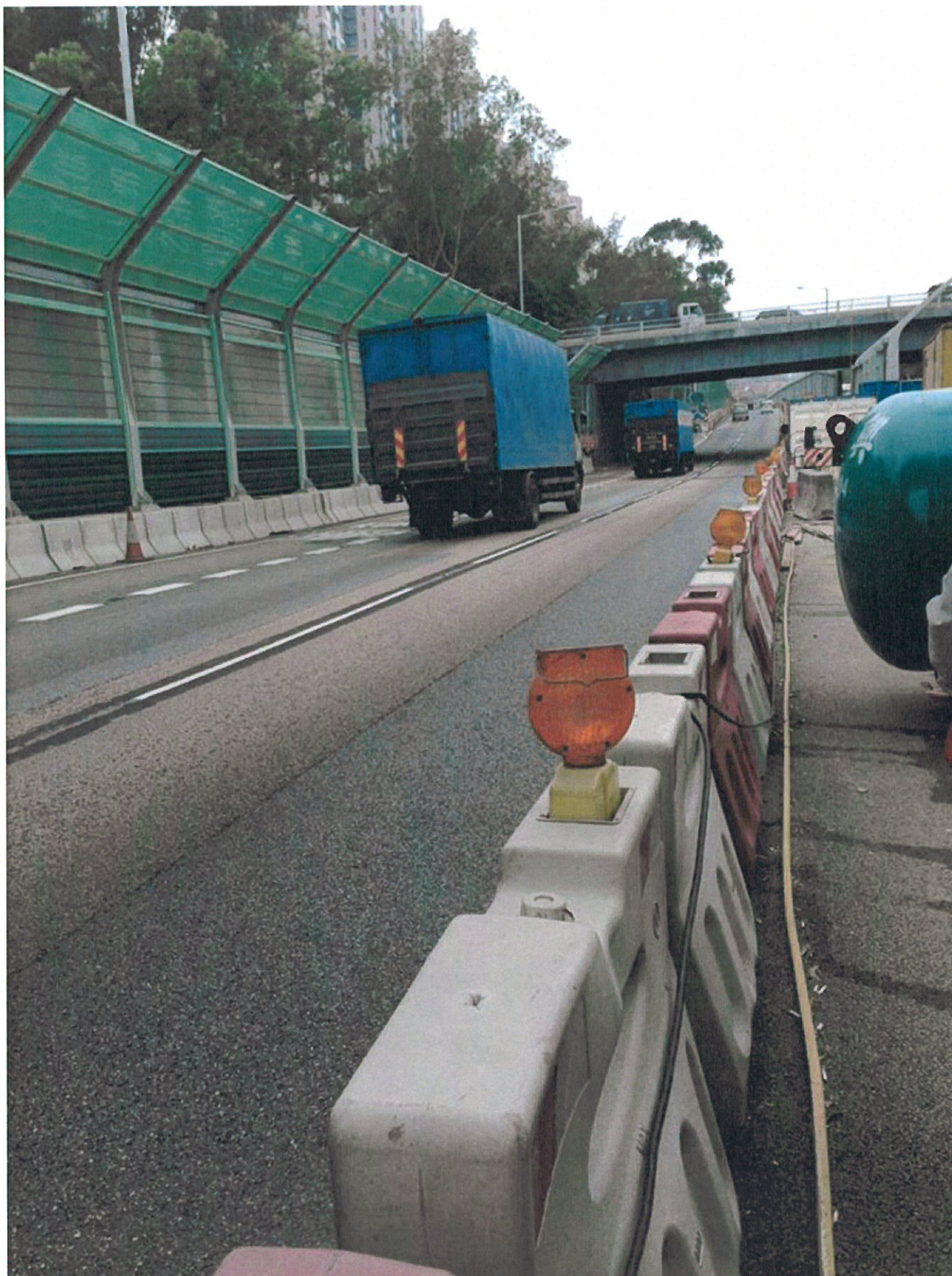
Figure 2 – The works area screened by existing noise barriers
