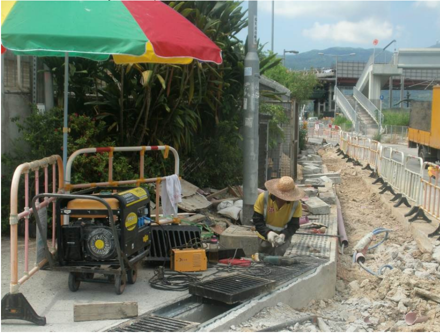
Photo 2: Excavated area and exposed earth near the monitoring location (Date: 23 July 2016)
