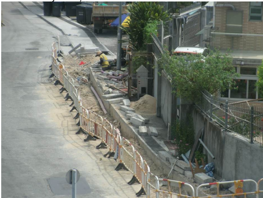
Photo 1: Road Works observed near the Air Quality Monitoring Station (Date: 23 July 2016)
