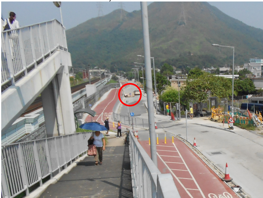
Photo 1: Excavation Site observed within proximity of SR77 (Red Circle) (Date: 17 October 2014)
