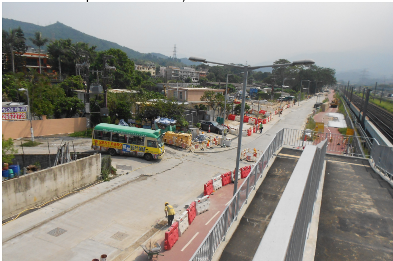
Photo 1: Construction area observed within proximity of SR77 (Date: 19 September 2014)
