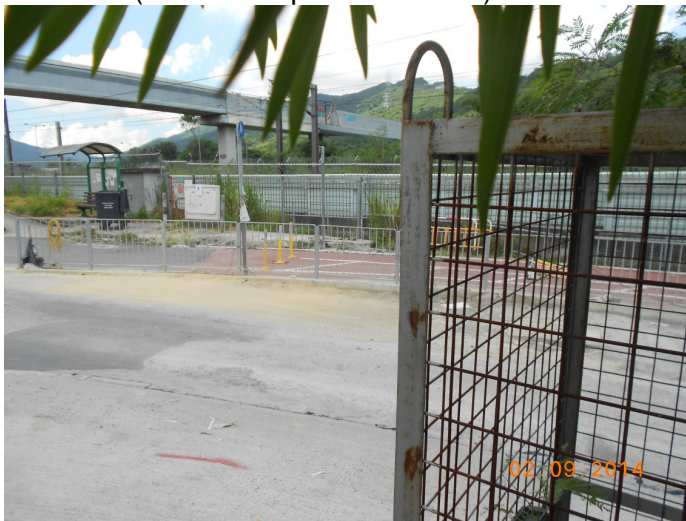
Photo 3: Dusty materials observed unattended within close proximity of SR77 (Date: 2 September 2014)
