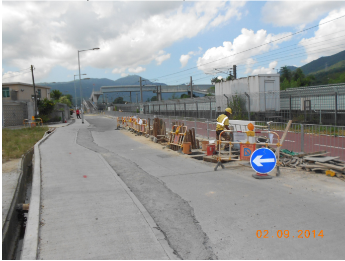
Photo 2: Construction works observed within close proximity of SR77 (Date: 2 September 2014)
