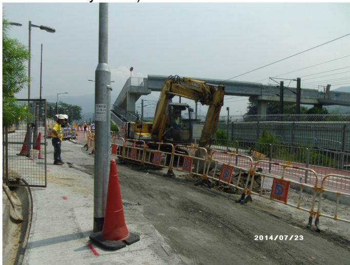
Photo 1: Construction works observed within close proximity of SR77 (Date: 23 July 2014)
