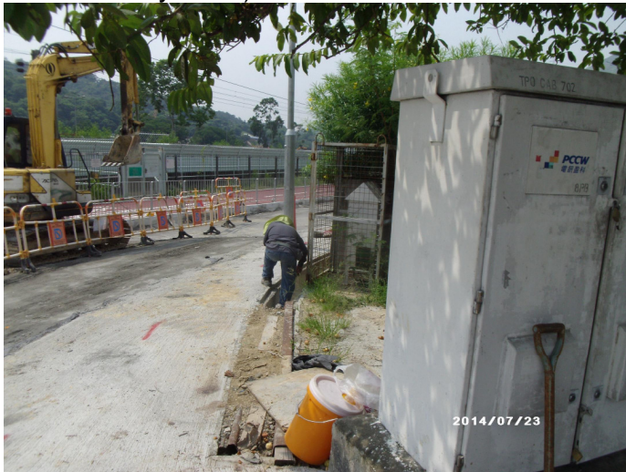
Photo 2: Construction works observed within close proximity of SR77 (Date: 23 July 2014)
