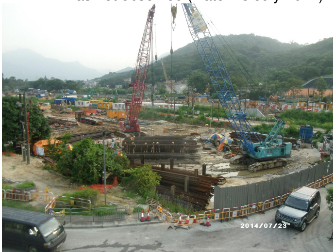
Photo 3: Overview of the construction works site which significant dust emission was not observed (Date: 23 July 2014)
