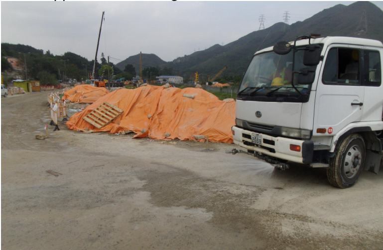
Dust suppression is being undertaken at construction site (Date: 24 March 2014)
