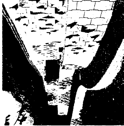
Series of re-inforced earth retaining walls adjacent to road with terracing and curved sculptural finish. Terrace areas may be planted with trees and shrubs.
